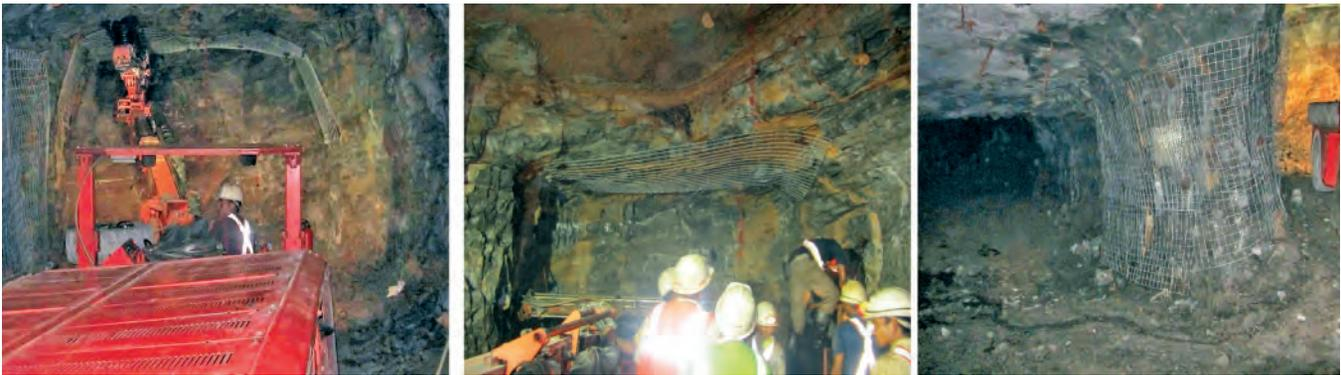
Fig.10 Fixation of welded support firmly to the immediate roof near the development face
