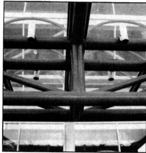
Fig. 1. Building entrance showing (left) overlapped and (right) non-overlapped connections
