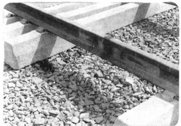
Fig 7 : Showing a good joint
