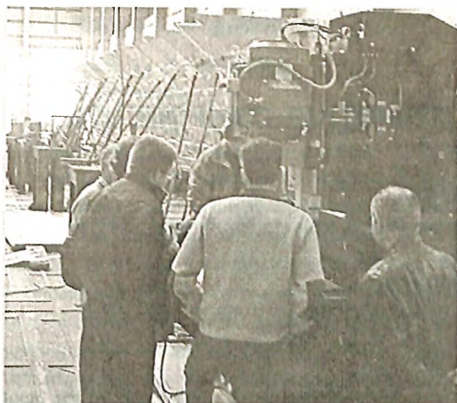
Figure - 4: FSW LEGIO™ 3UT installed next to shiphull production line at Estaleiros Navais do Mondego S.A. Shipyard in Portugal
