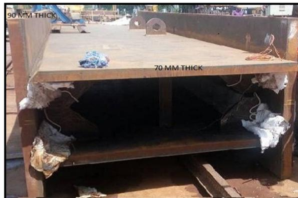
Fig. 2 : Assembled box with preheater
