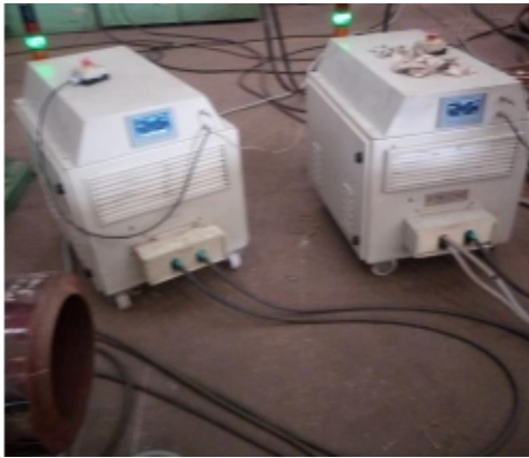
Fig. 4 : Two inter-locked controllers feeding two coils for PWHT at 750 deg C
