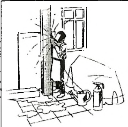
Fig. 8 : It is important to protect fire sensitive things where there is a risk of fire when welding
