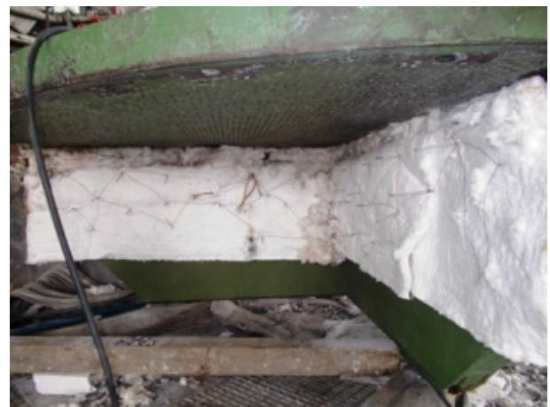
Fig. 2 : Showing Post Heating Arrangement of Sieve Plate after Weld
