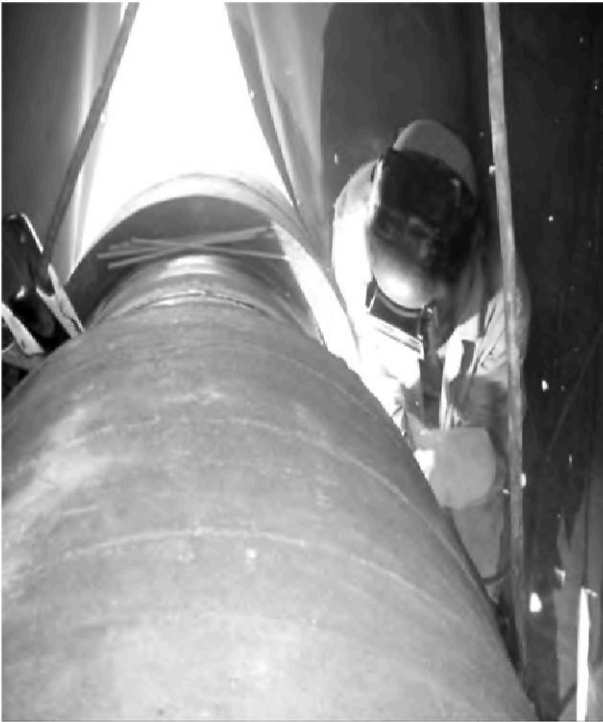
Application of PPE during welding
