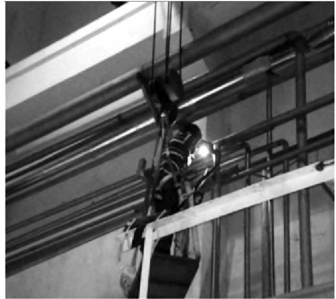
Fig. 8 : Welding of main LN 2 transfer line at 12 meter height
