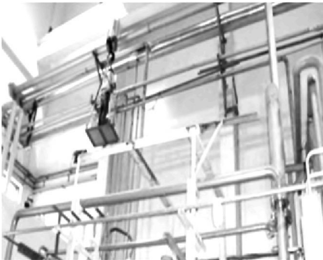
Fig. 11 : Repaired LN 2 line at 80 K
