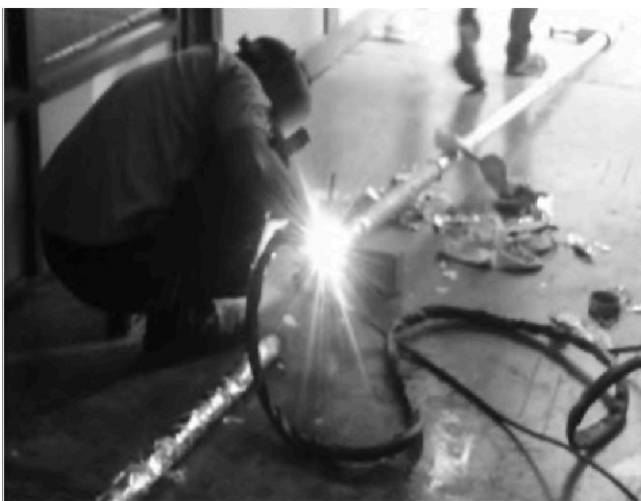
Fig. 7 : Welding of Bellows with transfer line
