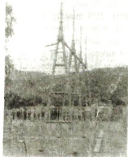
Fig 5 : 42 Tubular Structure Erected at Chamera H.E. Project
