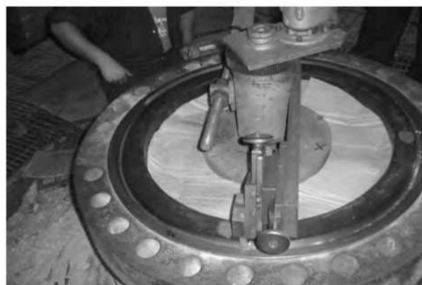
Fig. 3: In-situ machining at RTJ groove of man-way flange to remove cracks
