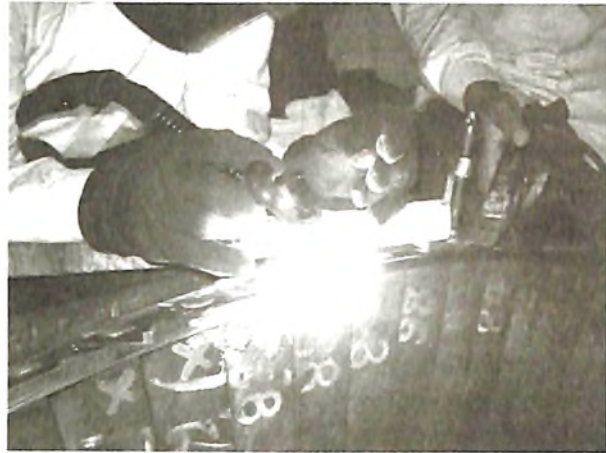
Fig. 5 : Photograph taken during welding of shroud piece
