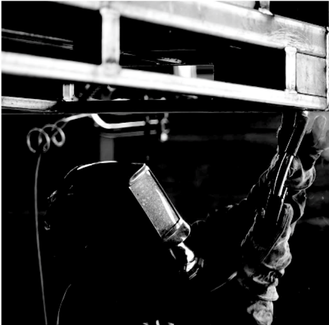
Fig. 1 – Like many manufacturers, Advanta Southeast has turned to automation to overcome the shortage of skilled welders.
