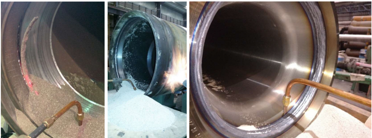
Fig. 6 : Sub arc welding of moulds and continuous heating of large moulds
