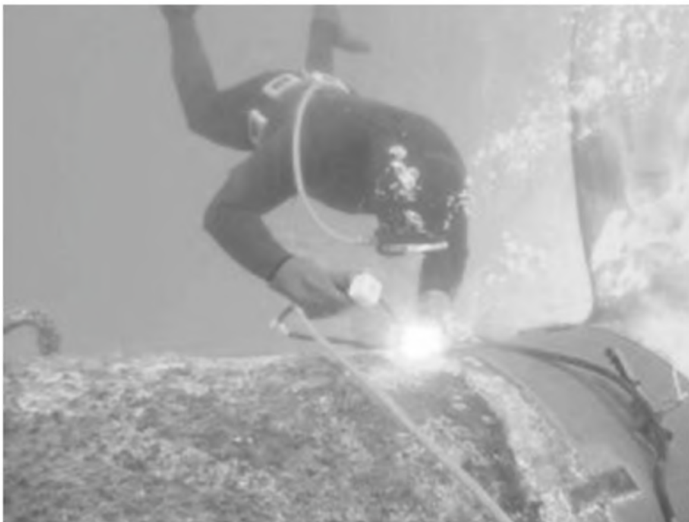
Fig. 3 : Wet underwater welding [6]
