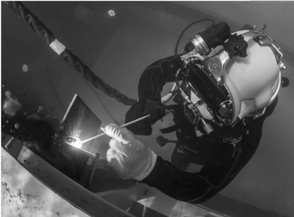
Fig. 4 : Wet underwater welding [7]
