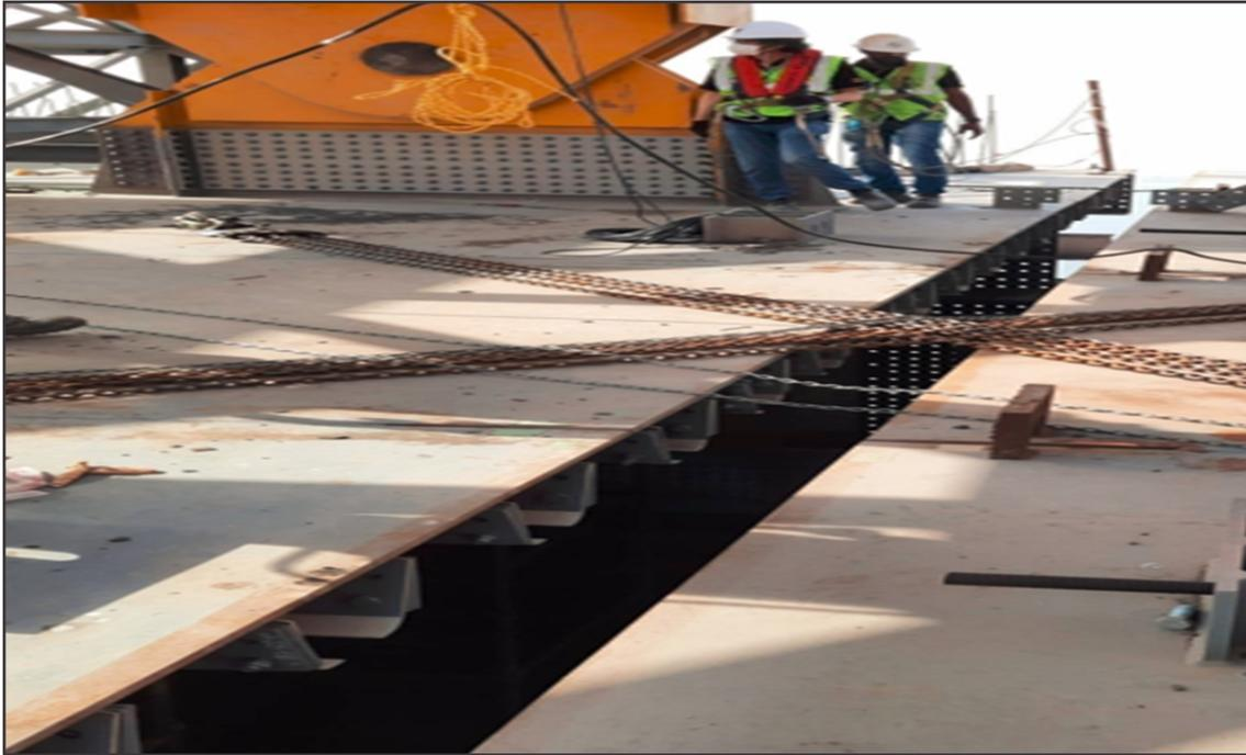
Fig. 22 : Locking of 2-meter span near fit-up area
