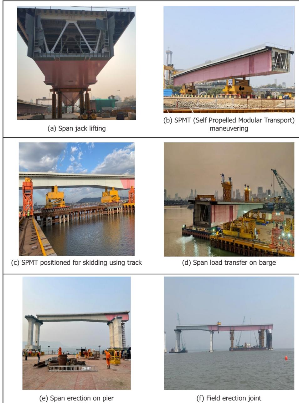
Fig. 18 : Stages of Span transportation from assembly yard to erection at marine location
