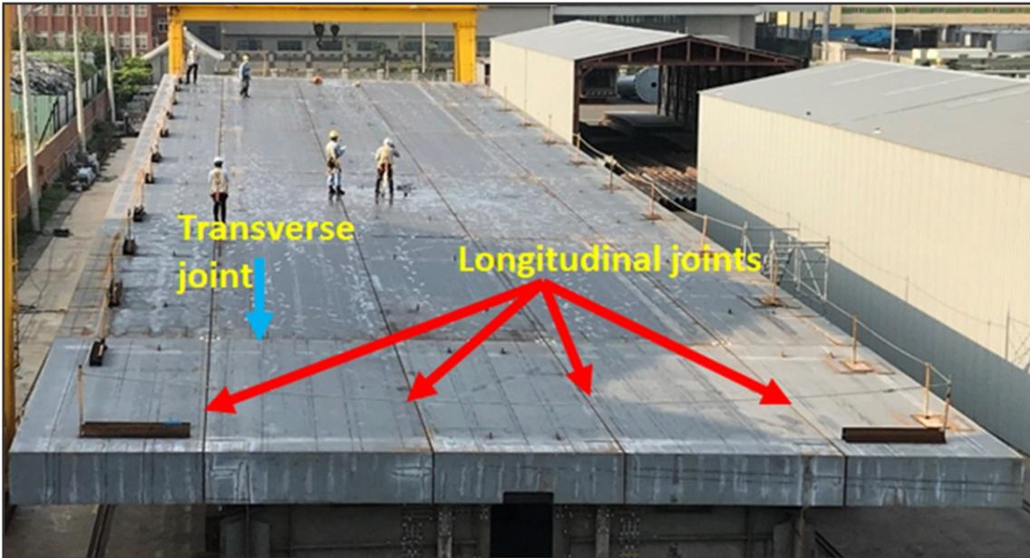
Fig. 4 : Span Assembly Showing Longitudinal and Transverse Joints
