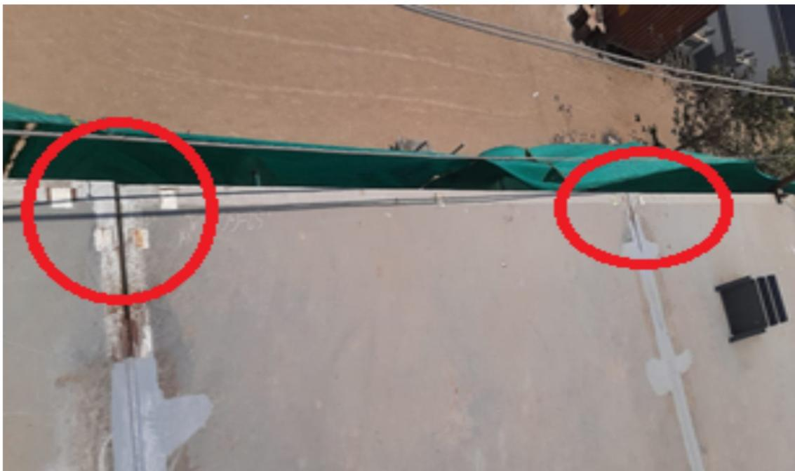
Fig. 14 : Un-welded portion(300mm) of longitudinal joints
