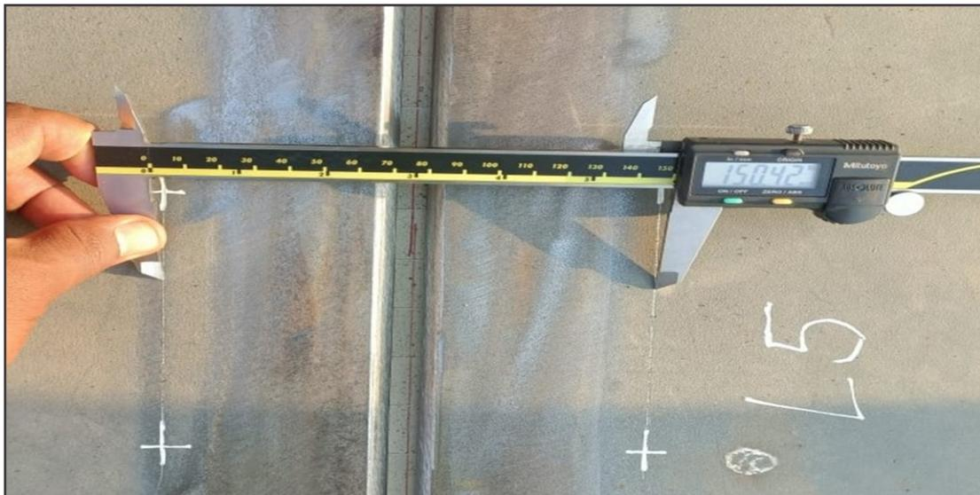
Fig. 21 : Measuring match marking 150mm before welding
