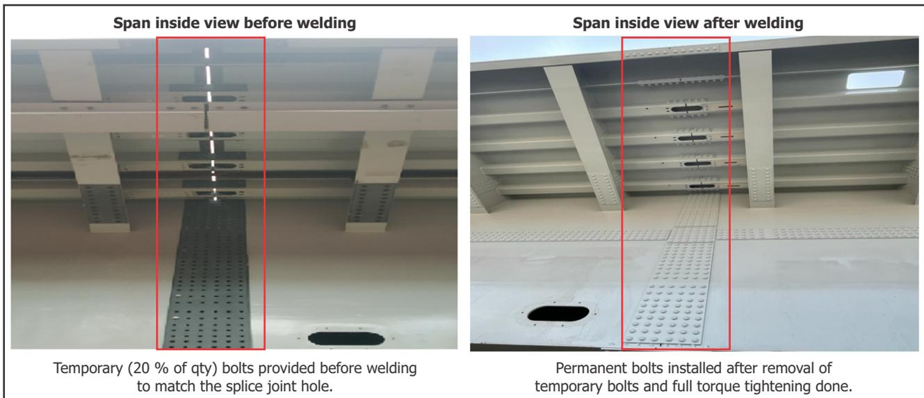
Fig. 12 : Bolt tightening before and after welding
