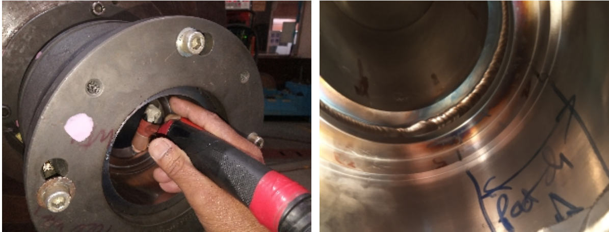
Fig. 10 : Welding at a difficult to access joint
