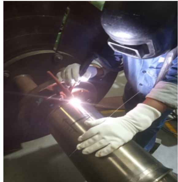
Fig. 8 : Welding in progress
