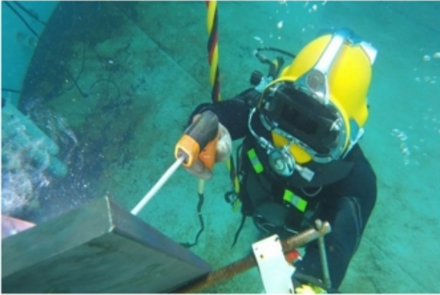
Fig. 3 : Wet Underwater Welding [10]
