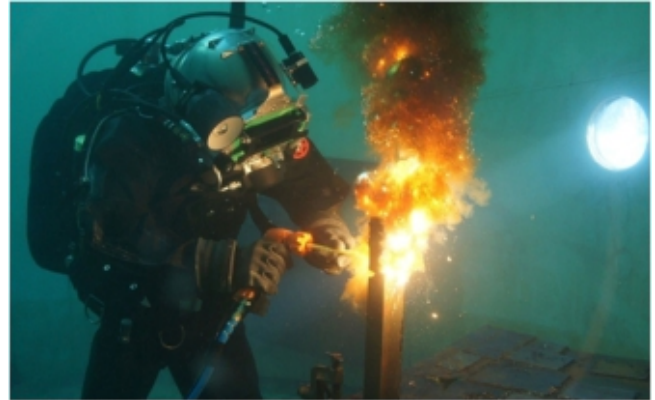
Fig. 5 : Gas formations and bubbles in Underwater welding [40]
