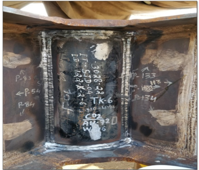
Fig. 3 : Sector tubular joints by FCAW
