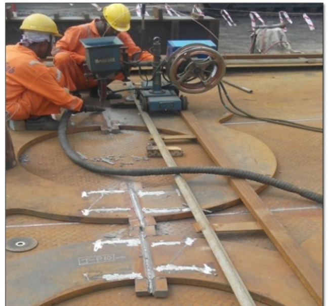
Fig. 4 : Details Plating joints by SAW
