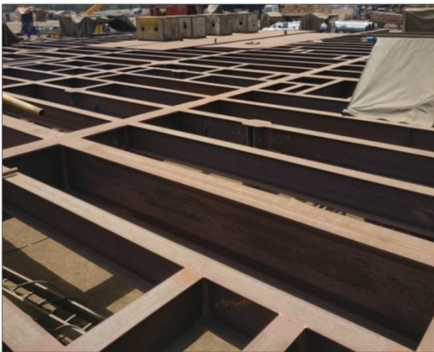
Fig. 2 : Framing beam (XYZ) joints by FCAW
