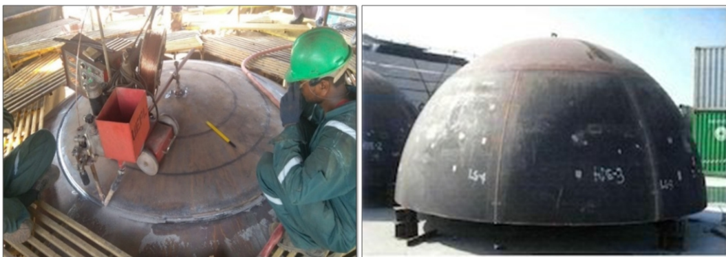
Fig. 10 : Welding using SAW with In-house arrangement
