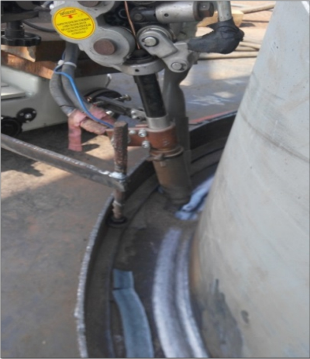
Fig. 1 : Framing Main Leg to detail Joints by SAW
