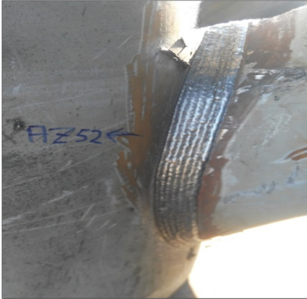
Fig. 5 : T-K-Y Joints by FCAW
