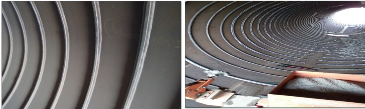
Fig. 9 : Shear Key Welding by SAW
