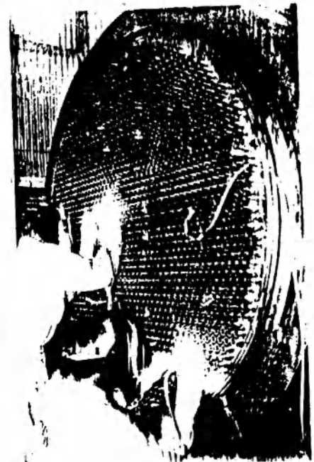
Fig 7 : Manual GTAW of Titanium Tube to Tubeheet on the job
