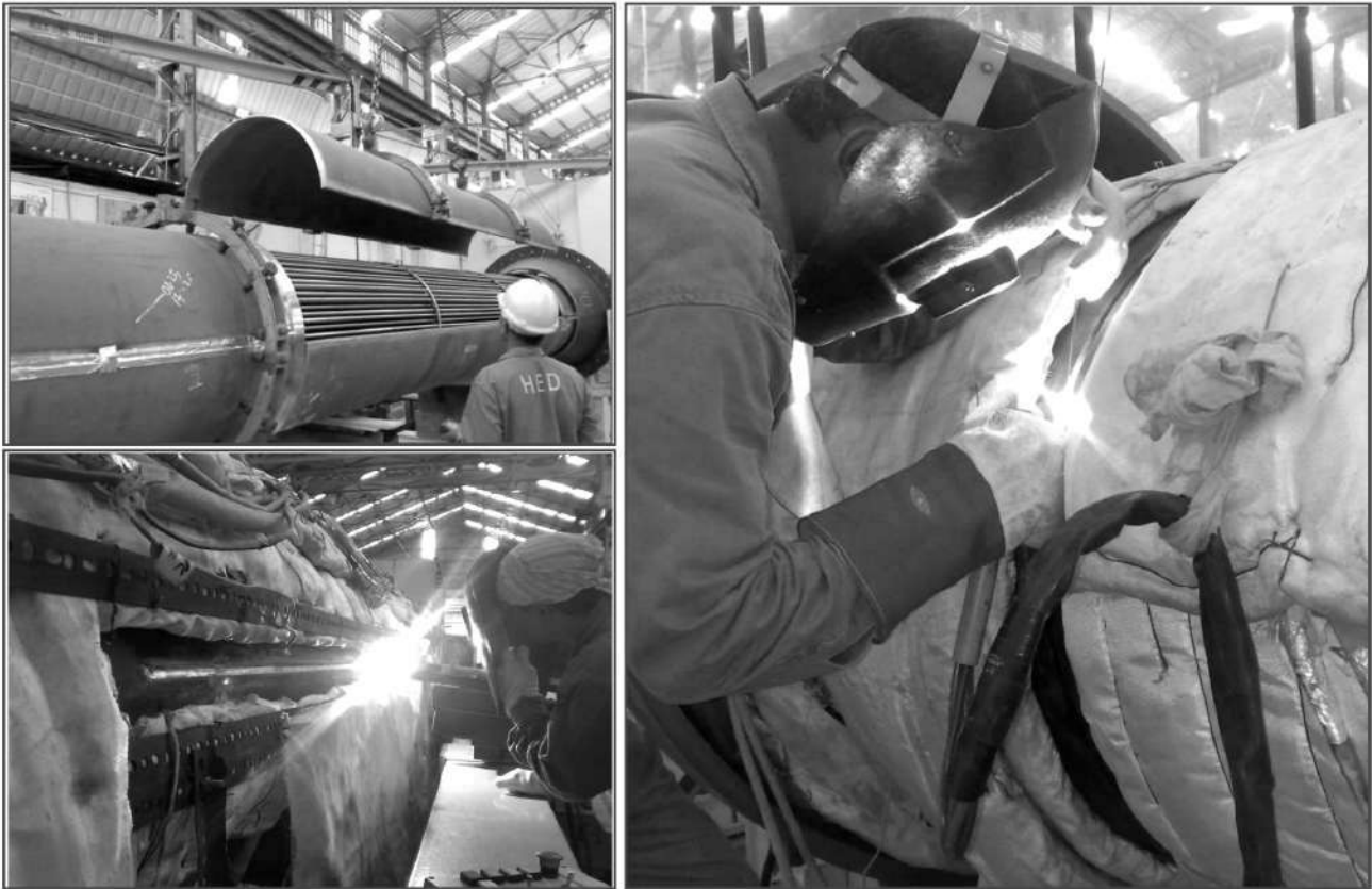
Fig. 2 : Shell welding of Steam Generator around the tube bundle
