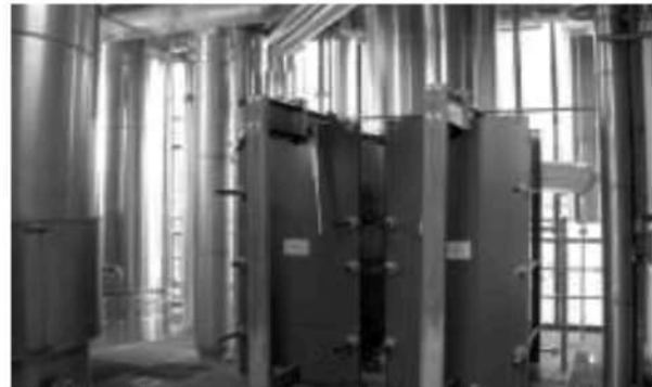
Fig.10 : Heat exchanger made out of Titanium Alloy
