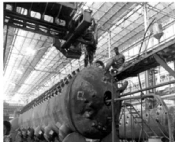
Fig. 23 : Tandem SAW of Boiler Drum Long Seam
