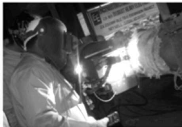
Fig. 16: Orbital Pipe Welding by RMD process
