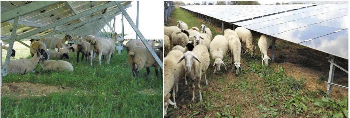
Fig.2: Agri-solar installations (courtesy: https://ratedpower.com/blog/benefits-agrivoltaics-examples/ )
