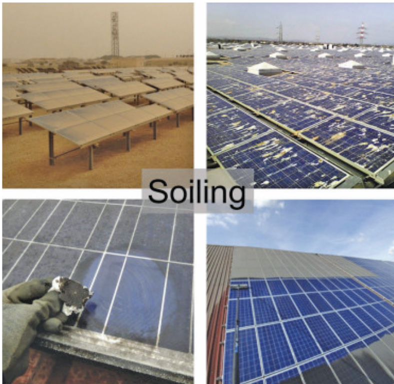
Fig.3: Soiling losses
