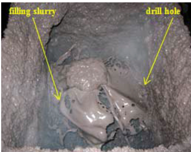
Fig.6 Pipeline transfer of filling slurry
