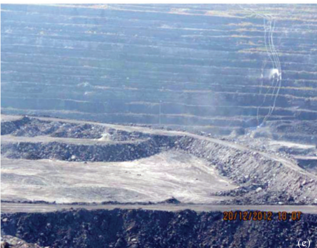
Fig.7 (a) Alternate layers of fly ash OB admixture and OB (b) Decks with fly ash as admixture in overburden material after compaction (c) Embankments constructed for backfilling the mine void
