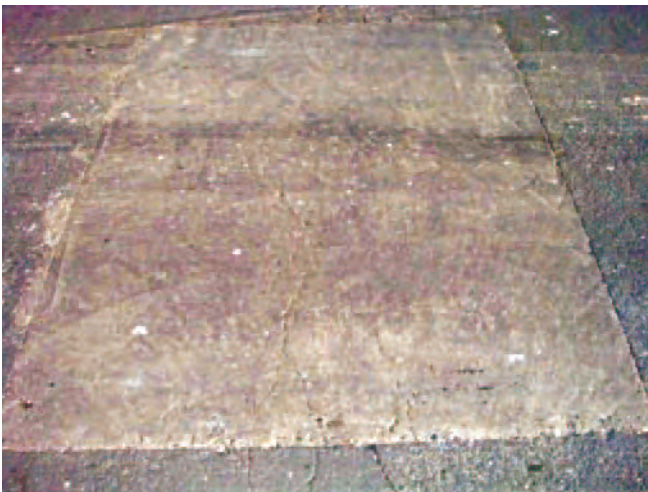
Fig.2 Repaired deck pavement
