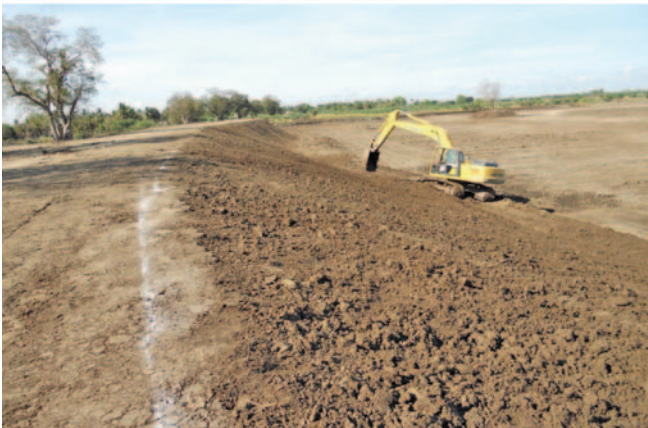
Fig.5 Walajah lake - de-silting work
