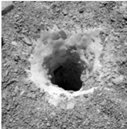
Fig.2 Screened drill cuttings used as stemming material used in charged holes
