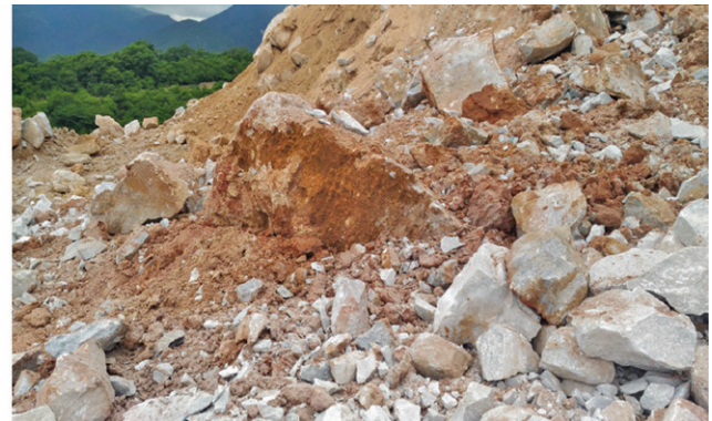
(b) Ineffective fragmentation of boulders in the face
