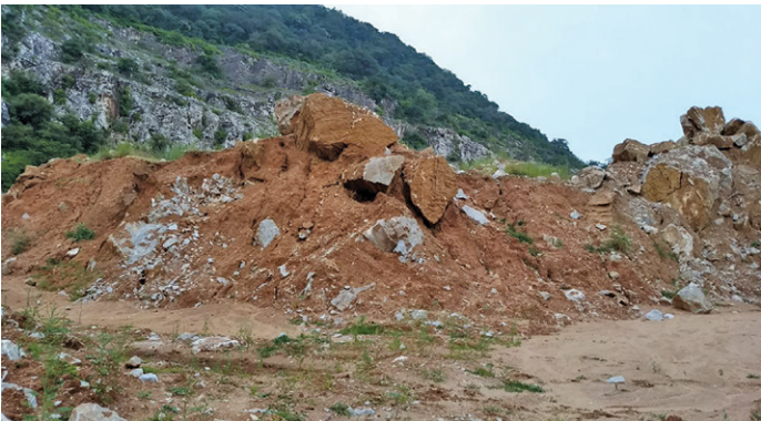
Fig.8: (a) Presence of embedded boulders in the face
