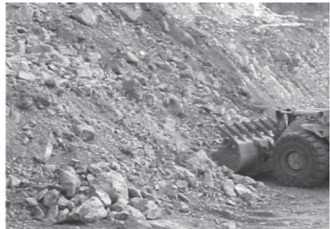
Fig.4 Blasted muck loading by FEL
