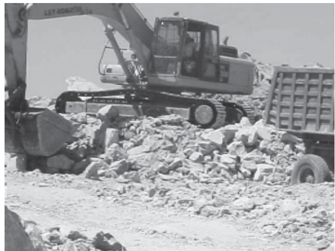
Fig.5 Backhoe struggling for loading muck
