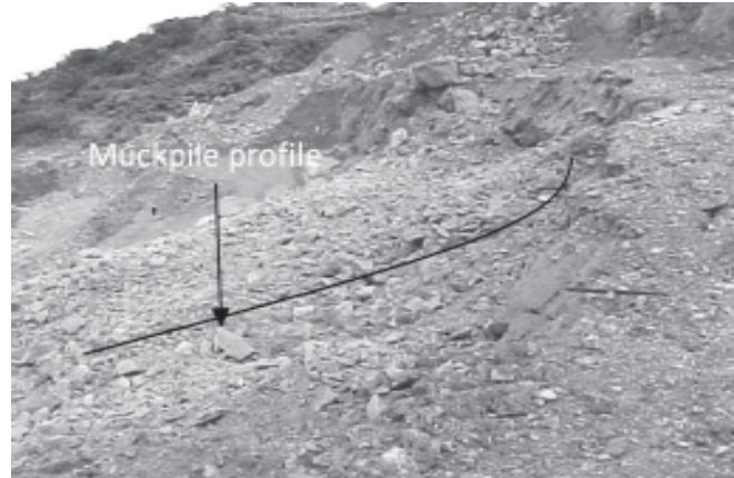
Fig.3 Good spreading of blasted muck
