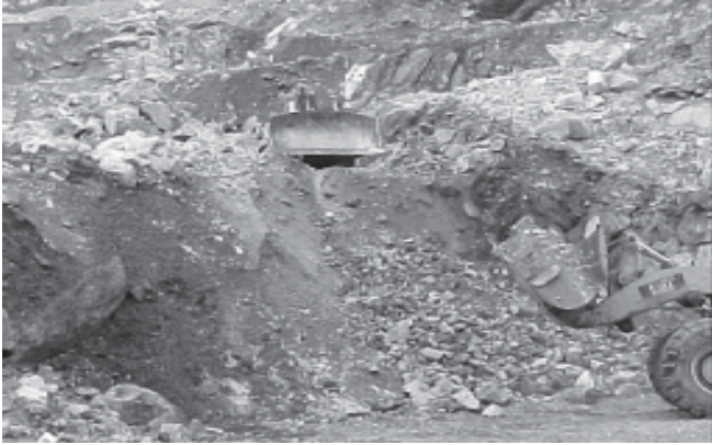
Fig.12 Compact, less spread muck loaded by FEL and dozer for support
