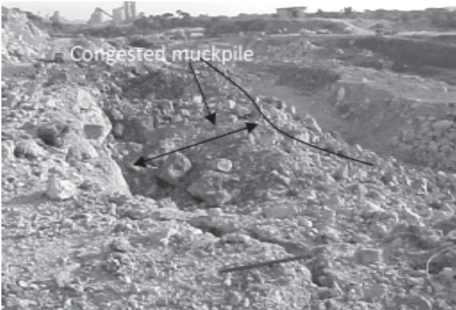
Fig.7 Congested, less spread blasted muck
