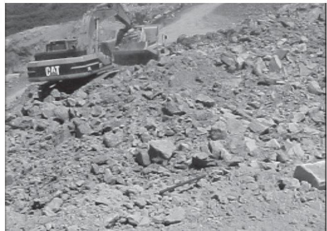
Fig.10 Blasted muck loaded by shovel
