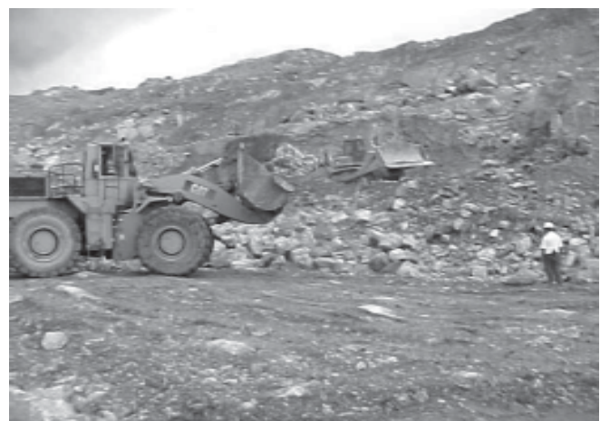
Fig.11 Bouldery muck loaded by FEL
