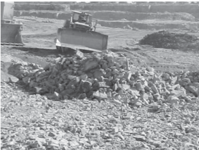
Fig.6 FEL collecting spread muck for shovel
