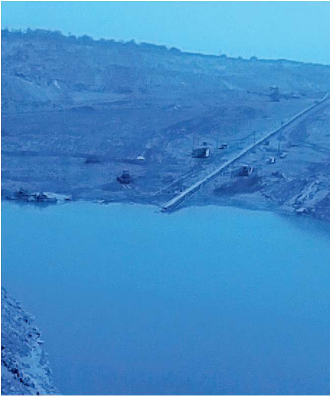
Fig.2 Current status of in-pit crusher and conveying system installed at PiparwarMine
