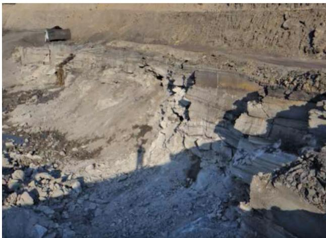
Fig.3 Joint planes parallel to highwall slope in T-3 (Bench: 0 to -6 m)
