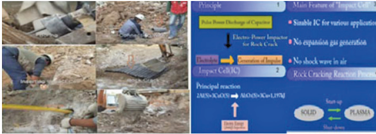
Fig.5 Rock breaking using plasma technology [14]
