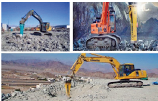
Fig.4 Application of hydraulic breaker
