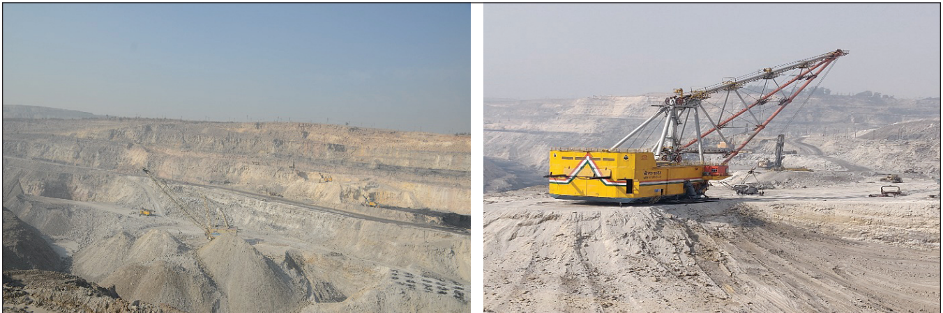
Fig.3: An overview of Khadia mines, NCL
