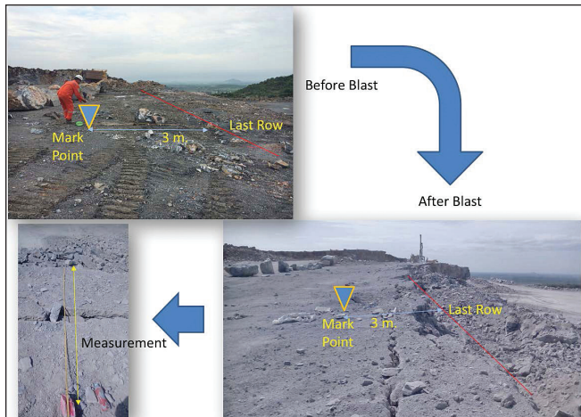
Fig.19: Backbreak measurement process after blasting
