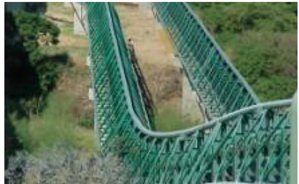
Typical “Triangular Gantry” structure
