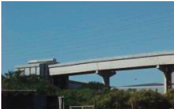
Typical “Concrete Gantry” structure
