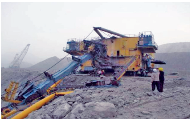
Fig.2 Draglineboom collapse in a large mine, India
