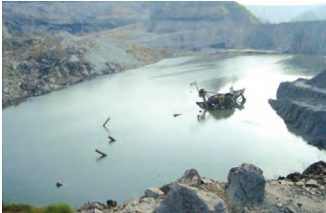
Fig.2 Regional failure of benches at Umrer OCP, WCL
