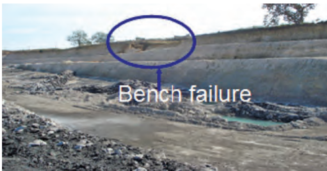
Fig.3 Local failure of bench at Dorli OCP-I, SCCL
