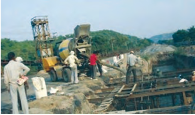
Fig.5 Civil foundation works
