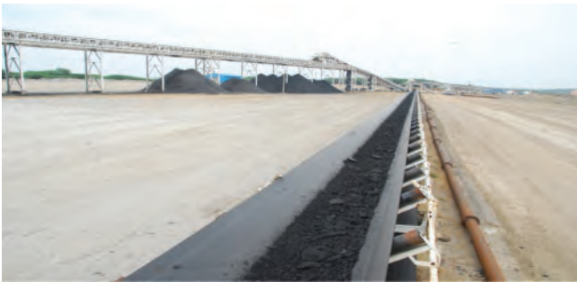
Fig.6 High capacity belt conveyor system
