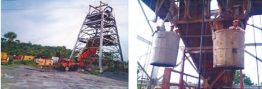
Fig.3(a) and (b) shaft sinking arrangements
