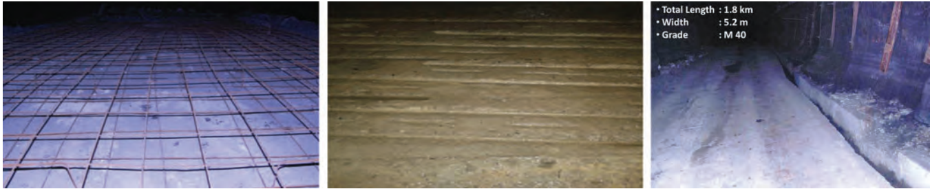
Fig.3(a) and (b) Construction of concrete roadway
