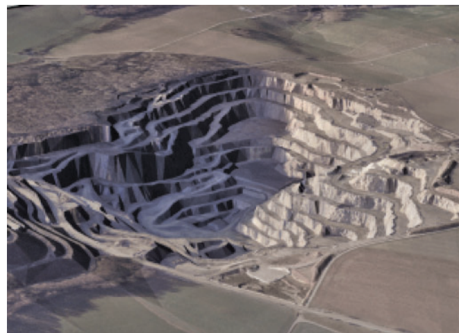
Fig.5 3D view at the open pit
