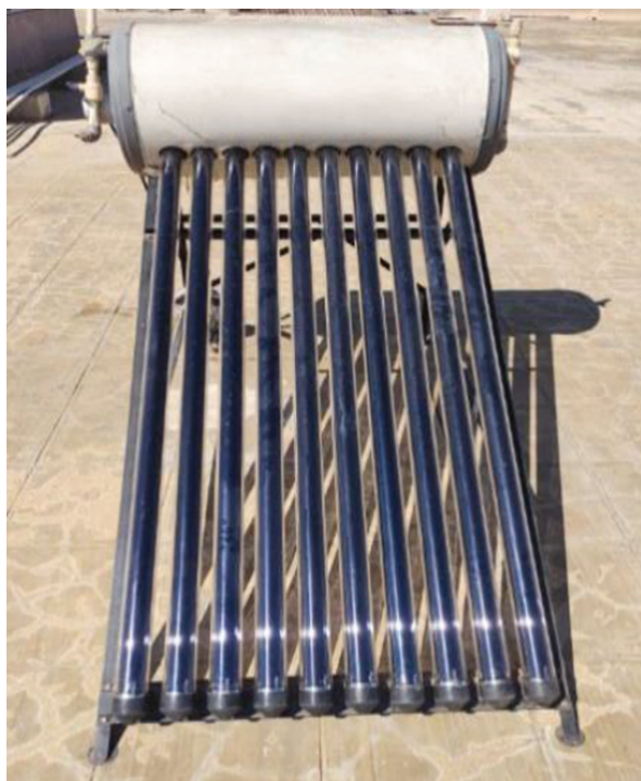
Figure 2: Solar water heating system
