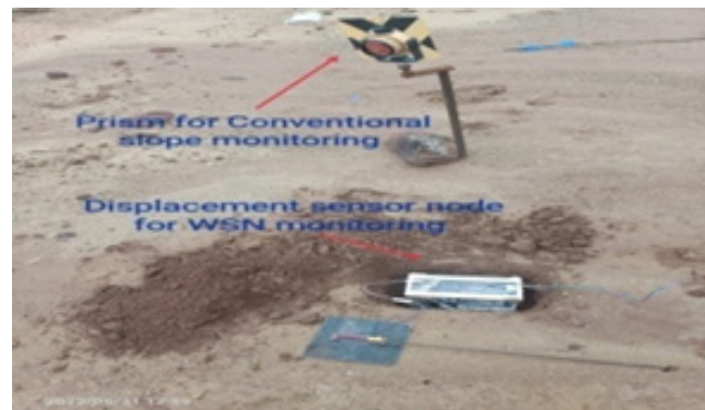
Figure 14. Fixing of deformation node in the 870 and 875 RL Benches.
