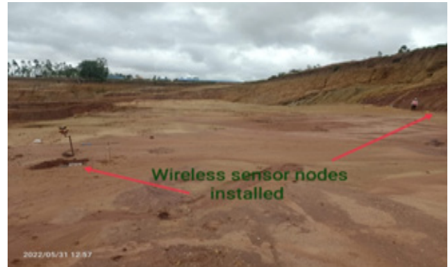
Figure 13. Location of monitoring points by installing the sensor nodes on the 870RL Bench.
