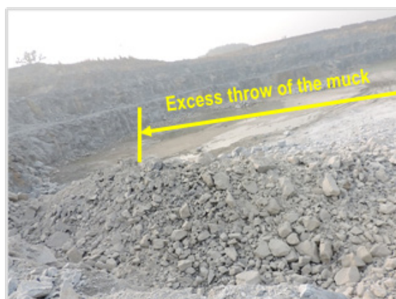
Figure 14. Excess throw of muck pile (diagonal firing pattern, LHS).
