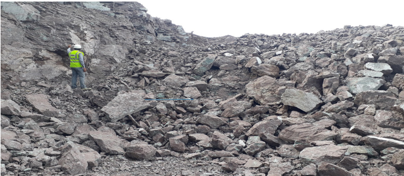
Figure 2. Muck profile achieved after blasting.
