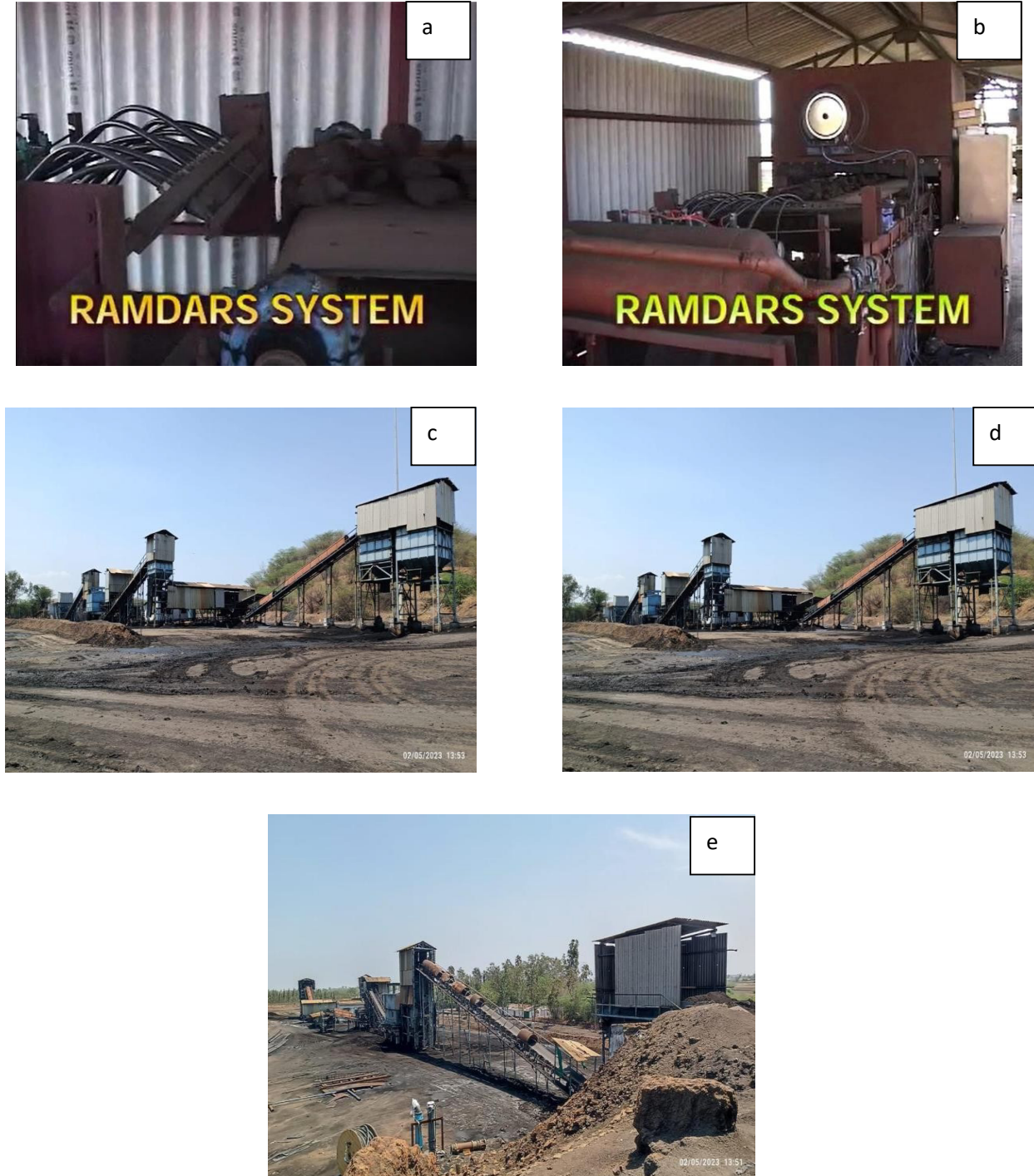
Figure 1. RAMDARS system installed in GHCL Bhavnagar Lignite deposits.
