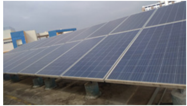
Figure 2. Installed 100 kW capacity grid connected polycrystalline PV system.
